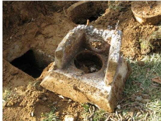
Typically the distribution box has failed as well due to age and corrosion
